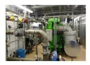
500kWe biogas CHP at RF Brookes, Newport
